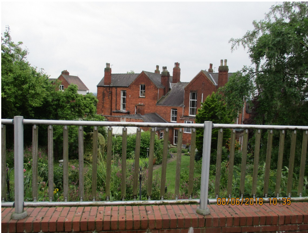
Looking to the rear of 129 Yarborough Road
