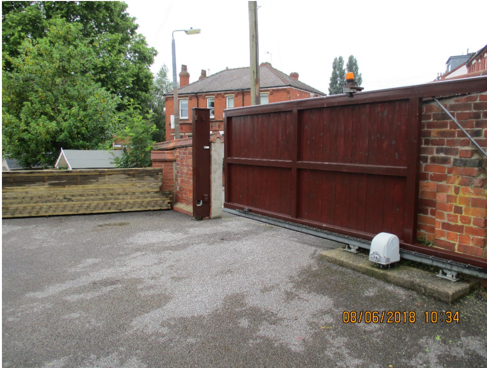
Within site looking at the auto gate
