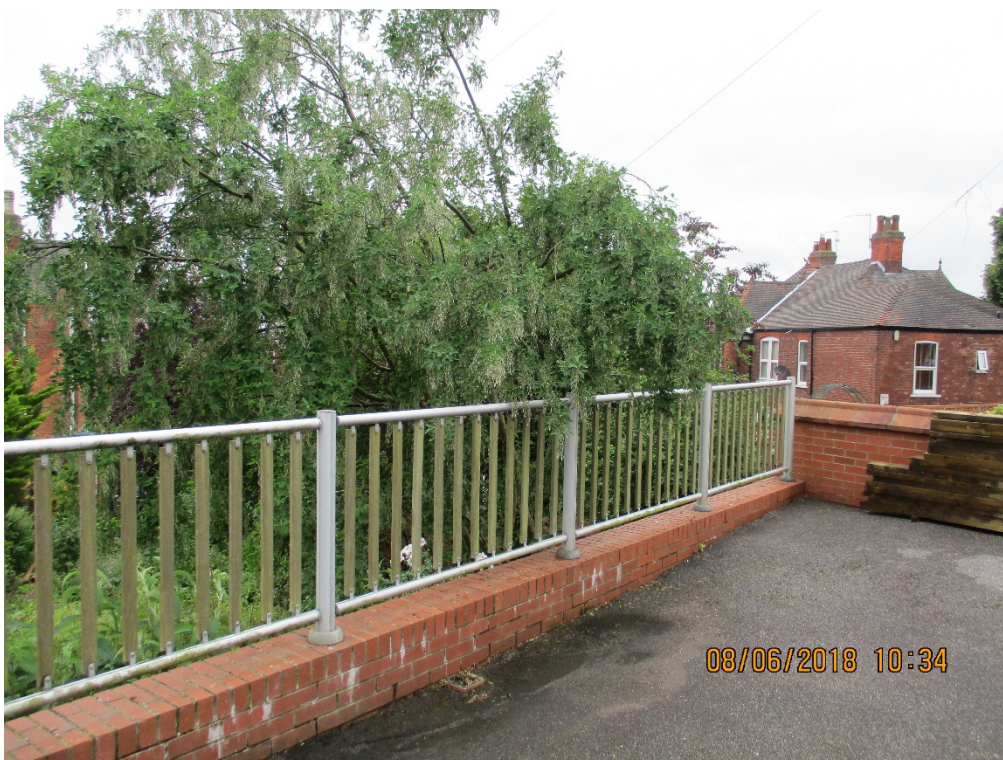
Looking to the rear of 131 Yarborough Road
